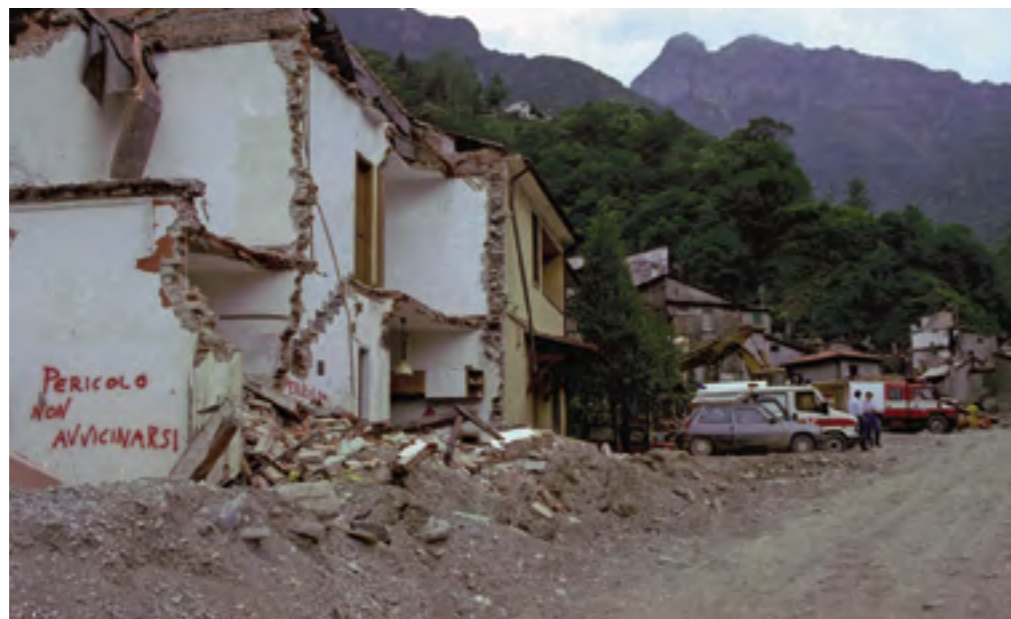
Photo 37. Houses destroyed in Versilia by the flood of 1996.
