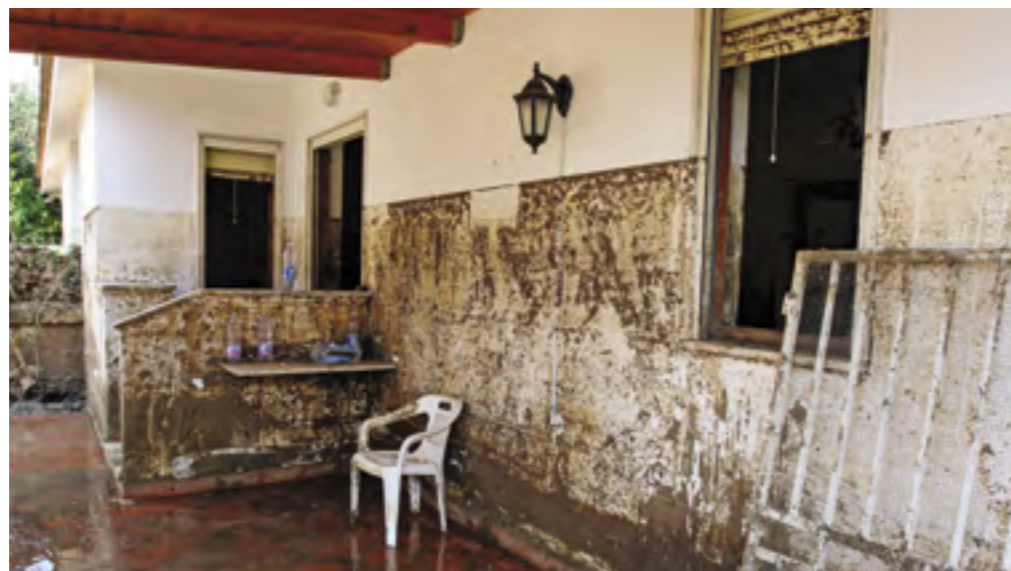
Photo 59. Vibo Valentia, 2006. House damaged by a flood.
