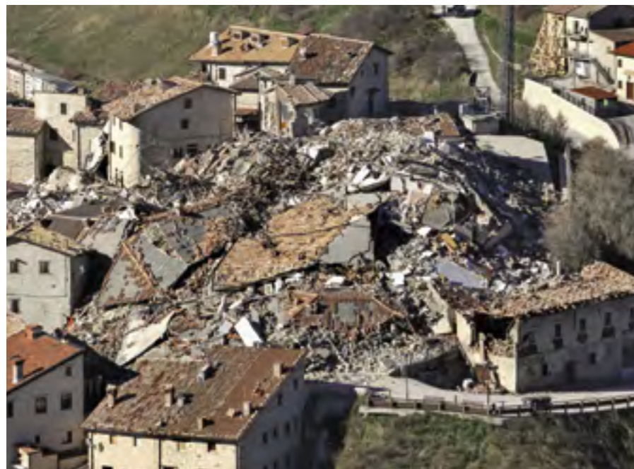
Photo 1. Castelluccio di Norcia, Perugia, 2016. Collapses caused by the 30 October earthquake.
