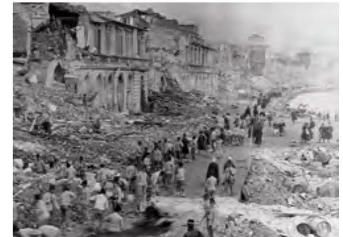
Photo 21. The devastating effects of the earthquake of 28 December 1908 in the city of Messina.
