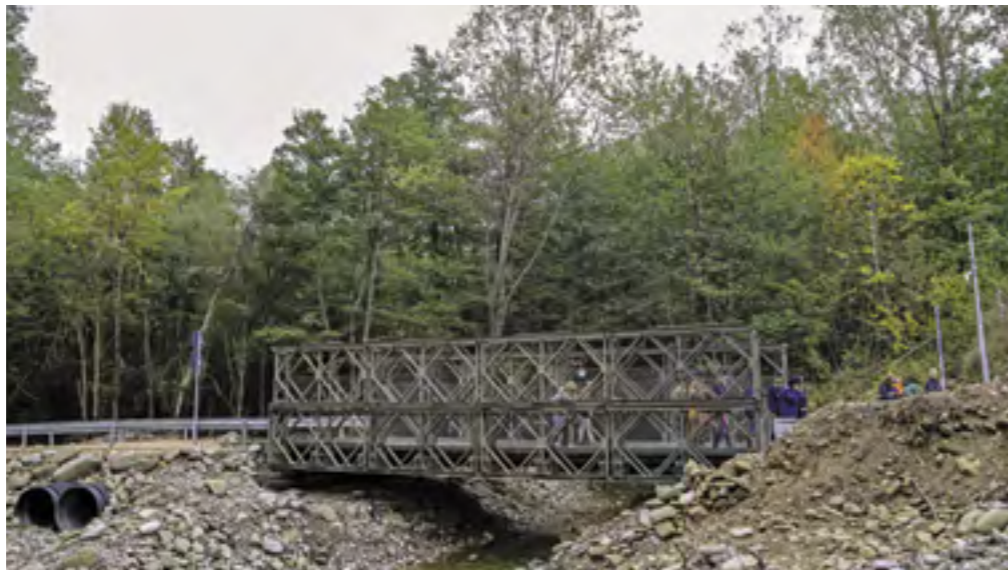
Photos 98, 99. Amatrice, 2016. Installation of a bailey bridge in Retrosi, to restore the road network.
