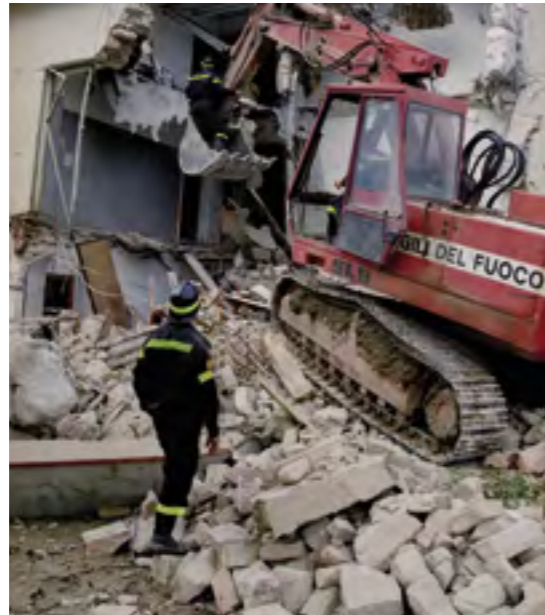
Photo 39. Damage to housing caused by the earthquake in Umbria and Marche.
