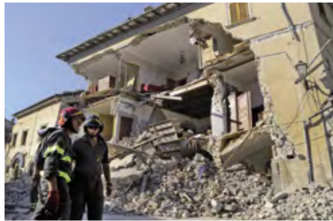
Photo 4. Amatrice, Rieti, 2016. Collapses caused by the 24 August earthquake.
