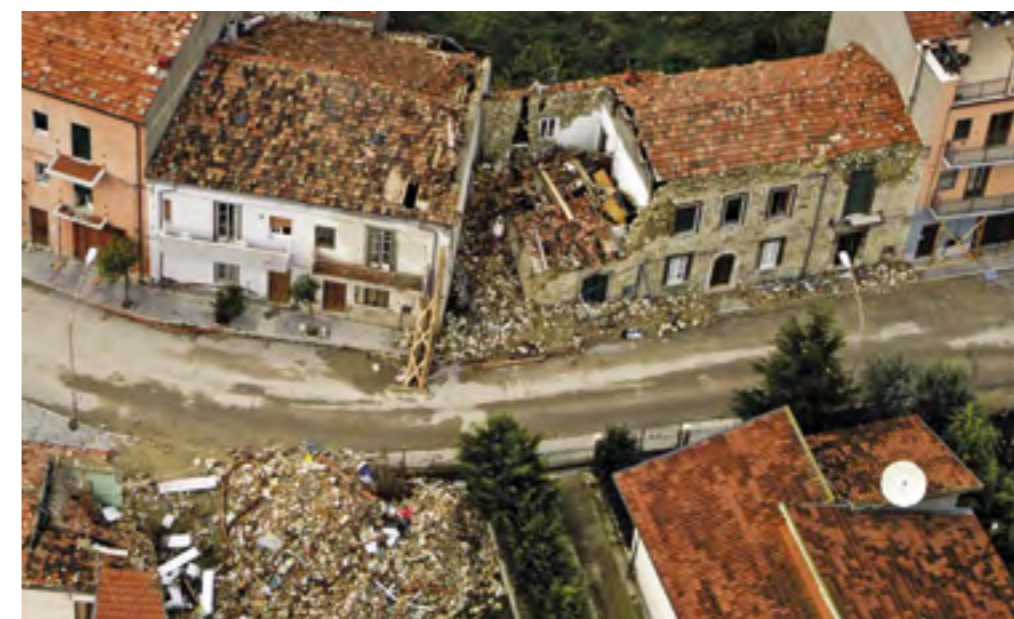
Photo 107. San Giuliano di Puglia, Campobasso, 2002. Collapses caused by the earthquake of 31 October.
