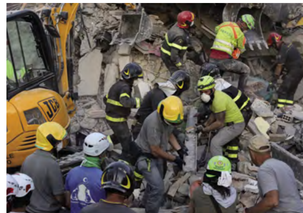
Photo 6. Amatrice, Rieti, 2016. Search and rescue activities after the 24 August earthquake.
