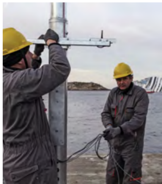
Photo 123. Giglio island, Tuscany, 2012. Technical experts at work in the shipwreck area of the Costa Concordia cruise ship.
