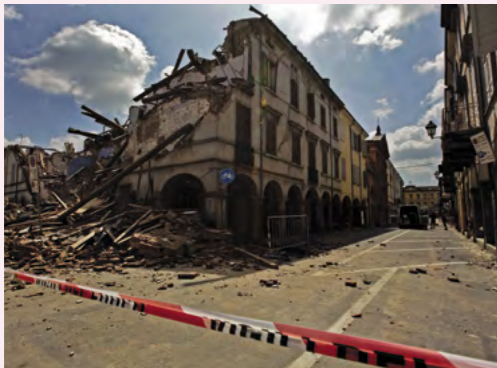
Photo 58. Concordia sulla Secchia, Modena, 2012. Damage caused by the 20 May earthquake.
