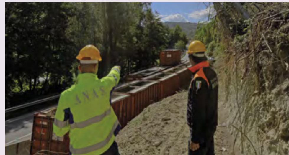
Photo 49. Pescara del Tronto, Ascoli Piceno, 2016. Mobility infrastructure restoration intervention following hydrogeological events triggered by the Central Italy earthquake.
