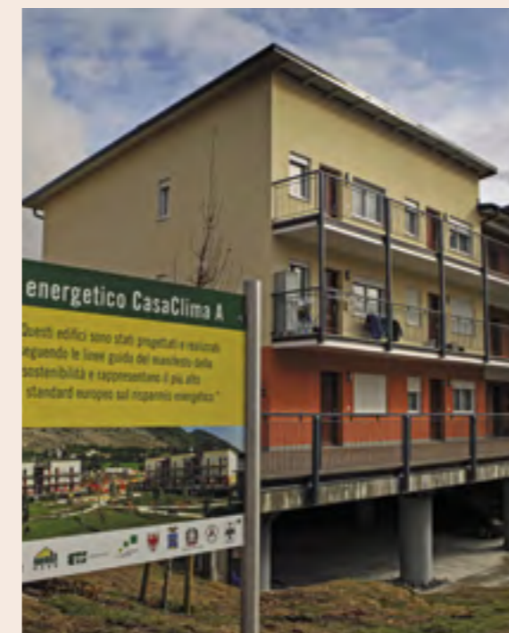
Photo 92. L'Aquila, 2009. House built within the framework of the CASE Project-Antiseismic Sustainable Eco-friendly Complexes.
