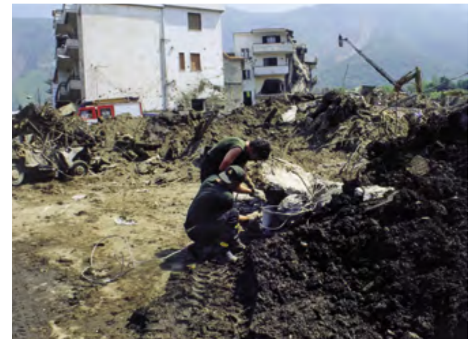
Photo 41. Sarno landslide of May 1998.
