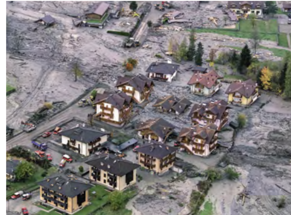
Photo 2. Dimaro, Trento, 2018. Building damage caused by an exceptional wave of bad weather.
