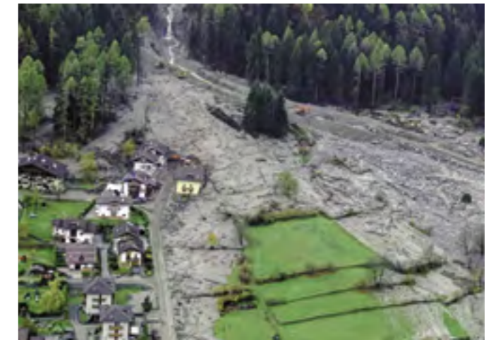
Photo 112. Trento, 2018. Damage to homes caused by an exceptional wave of bad weather.
