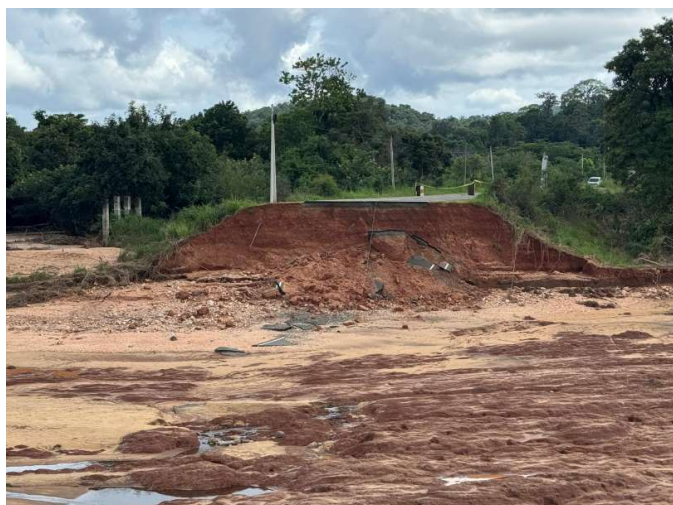
Photo 2 – Damage to embankment and right abutment completely exposed.
