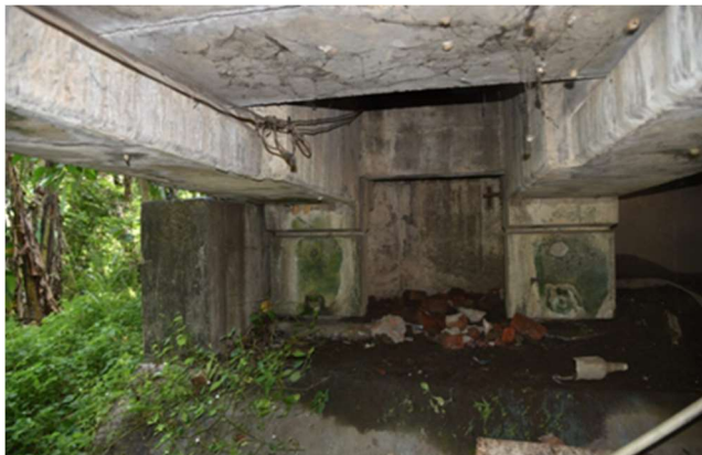
Photo 2 – Detail of the bearings on the piers/abutments cap
