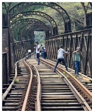
Photo 2 – Rotation of the pier (left), deviation of the rail (central and right).
