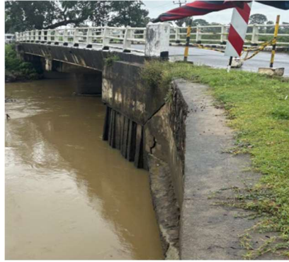
Photo 2 – Damage to the wing wall
