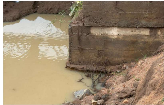
Photo 2 – Damage to the abutments
