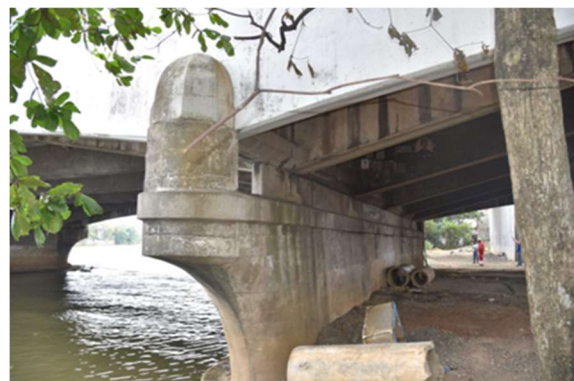
Photo 2 – Detail of the main girders (left) and pier cap (right).
