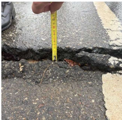
Photo 3 – Damage in proximity of the abutment (left) - 3D-modelling throw drone survey and assessment of the damaged area (right)
