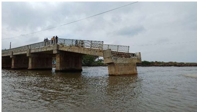
Photo 2 – View of the bridge section affected by the collapse
