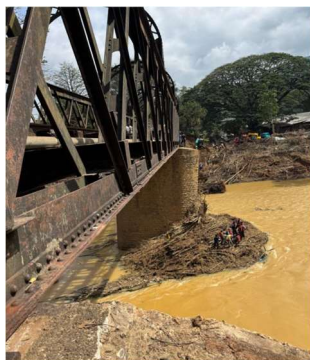
Photo 2 – Rotation of the pier (left), deviation of the rail (central and right).
