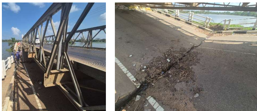
Photo 2 – View of the Bailey bridge (left), view of the bridge collapsed at the central pier (right).
