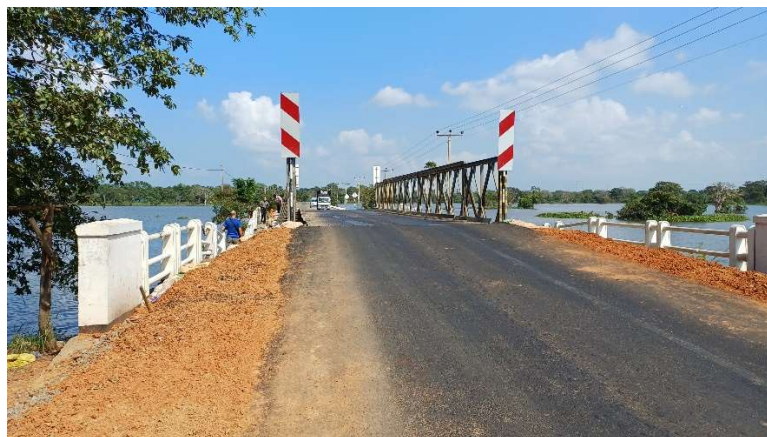
Photo 1 - View of the the bridge alignment and the temporary Bailey bridge.
