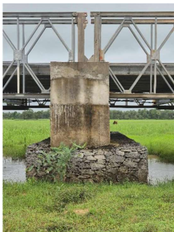
Photo 2 – Views of the rock caissons and abutments foundations
