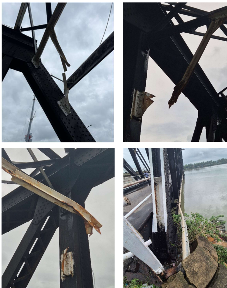
Photo 2 – View of damage to the diagonal bracing members and general conditions of the abutment
