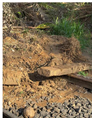
Photo 2 – Detail of landslide affecting railway tracks (left and center) and existing stabilization intervention (right)
