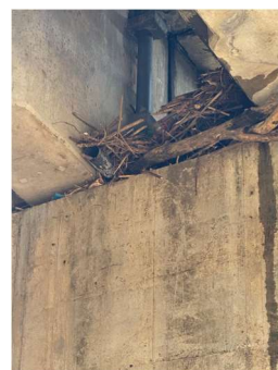
Photo 2 – debris on the foundation (left) and flow debris close to the bearings (right).
