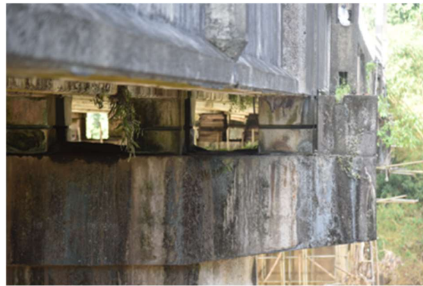
Photo 3 In the background the work (temporary bearings) on the central pier cap and on the right side the scaffolding with debris
