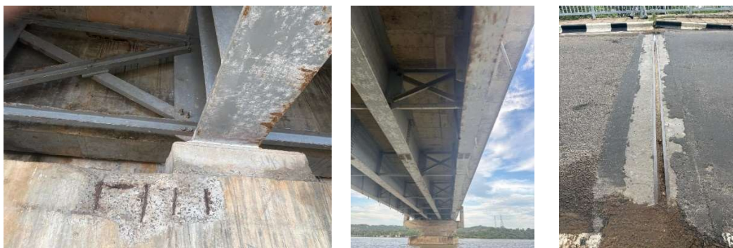
Photo 2 – Details of the corroded elements (left, central), detail of the joint (right).
