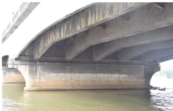
Photo 2 – Detail of the main girders (left) and pier cap (right).
