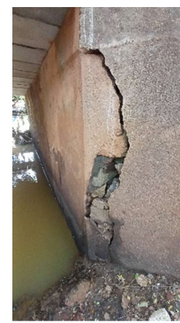
Photo 2 – View of the bridge deck soffit and riverbed with obstructive debris accumulation and damage to left abutment (left), and visible cracks between abutments and wing walls (central, right).
