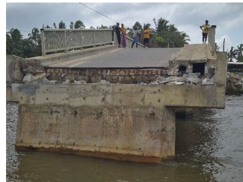
Photo 2 – View of the bridge section affected by the collapse
