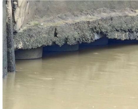
Photo 2 – Damage to the wing wall
