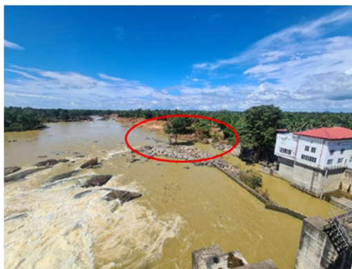
Photo 2 – View of the riverbed with indication of the damaged right bank
