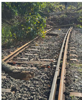
Photo 2 – Detail of landslide affecting railway tracks (left and center) and existing stabilization intervention (right)
