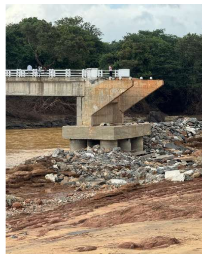
Photo 2 – Damage to embankment and right abutment completely exposed.
