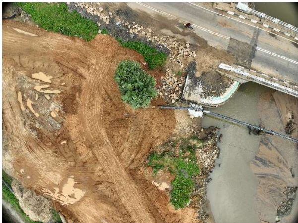
Photo 2 –View of damaged abutment to wing wall
