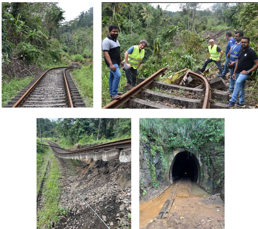
Photo 2 – Detail of first (upper left), second (upper right), third (lower left) landslide and tunnel 09 impacted by debris (lower right).
