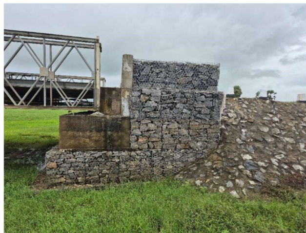
Photo 2 – Views of the rock caissons and abutments foundations
