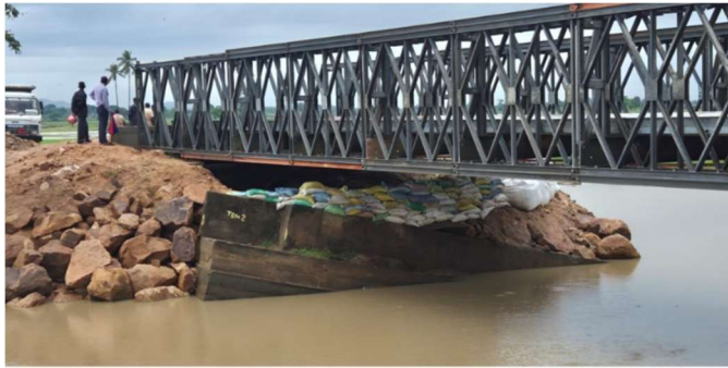
Photo 2 – Damage to the abutments
