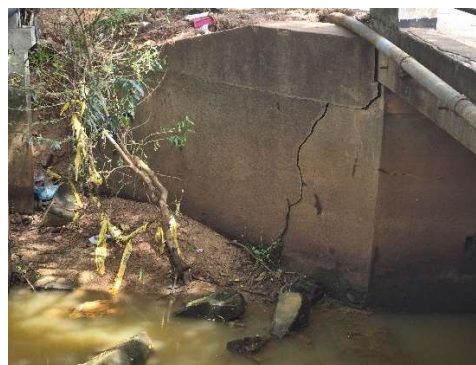
Photo 2 – View of the bridge deck soffit and riverbed with obstructive debris accumulation and damage to left abutment (left), and visible cracks between abutments and wing walls (central, right).
