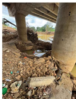
Photo 2 – debris on the foundation (left) and flow debris close to the bearings (right).
