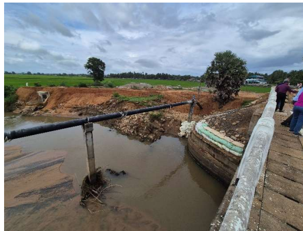
Photo 2 –View of damaged abutment to wing wall
