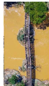
Photo 2 – Rotation of the pier (left), deviation of the rail (central and right).
