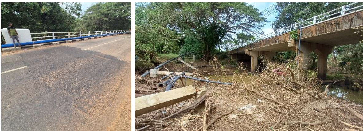
Picture 2 - View of the bridge from the left abutment, showing the repaired sinkhole (left), and the general condition of the riverbed after the flood (right).
