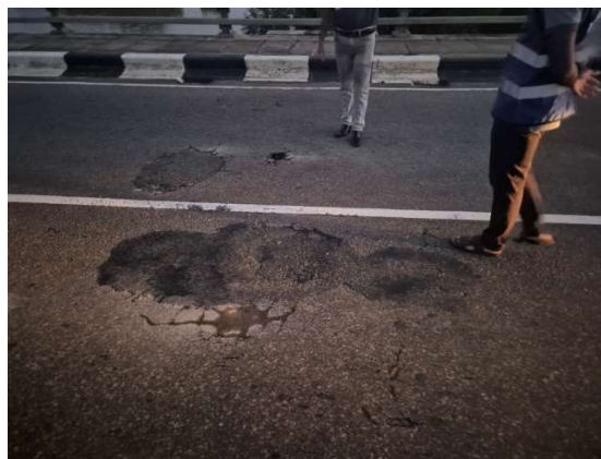
Photo n.2 – View of damage to the asphalt pavement.
