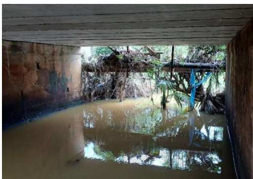
Photo 2 – View of the bridge deck soffit and riverbed with obstructive debris accumulation and damage to left abutment (left), and visible cracks between abutments and wing walls (central, right).
