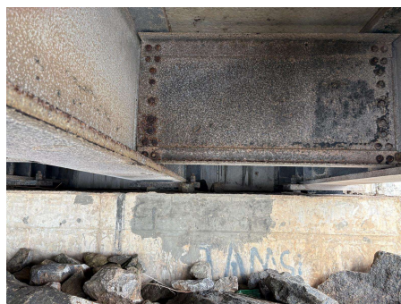
Photo 2 – Asphalt joints accommodating surface vibrations (left); corrosion of the deck steel frames (centre); corrosion of the pedestrian parapet (right).
