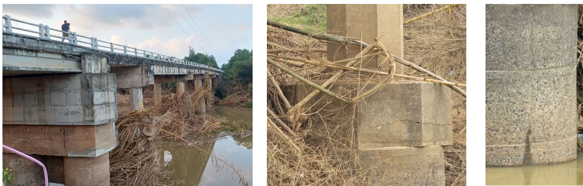
Photo 2 – View of the vegetative debris (left), details of cracks on foundation elements (central, right).
