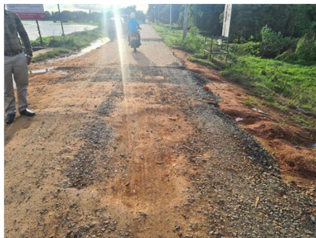
Photo 2 – View of the natural saddle surface erosion
