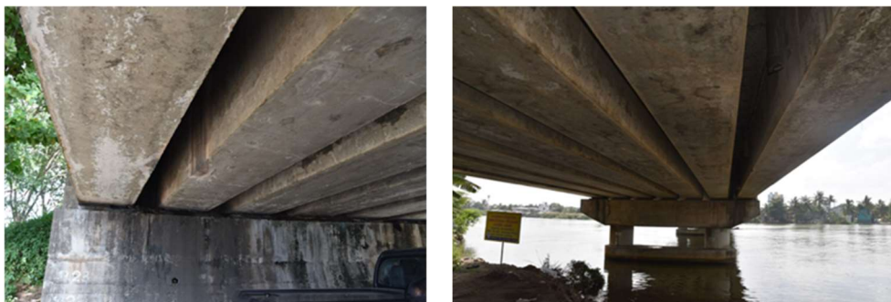
Photo 2 – Detail of underside of the deck and abutment (left) and pier (right).
